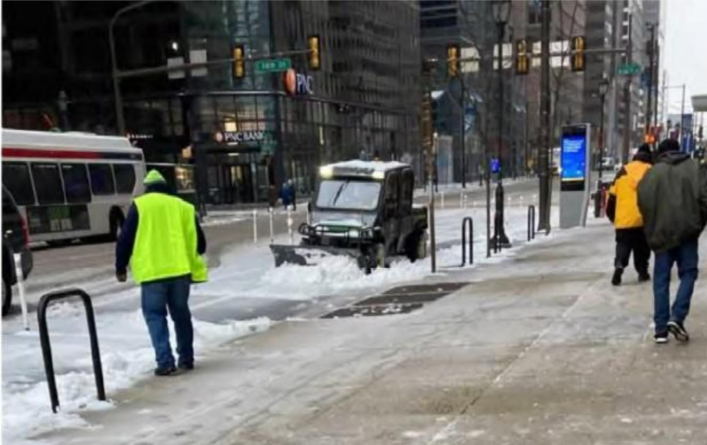
*Photograph 4:* Market Street, Philadelphia – Winter maintenance in Philadelphia. Smaller machinery utilized to minimize damage to delineator posts.
