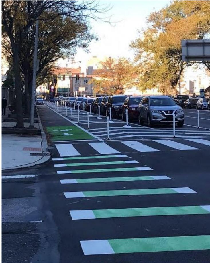
*Photograph 2:* Race Street, Philadelphia - Improvements include flexible delineators, striping, markings, and intersection treatment
