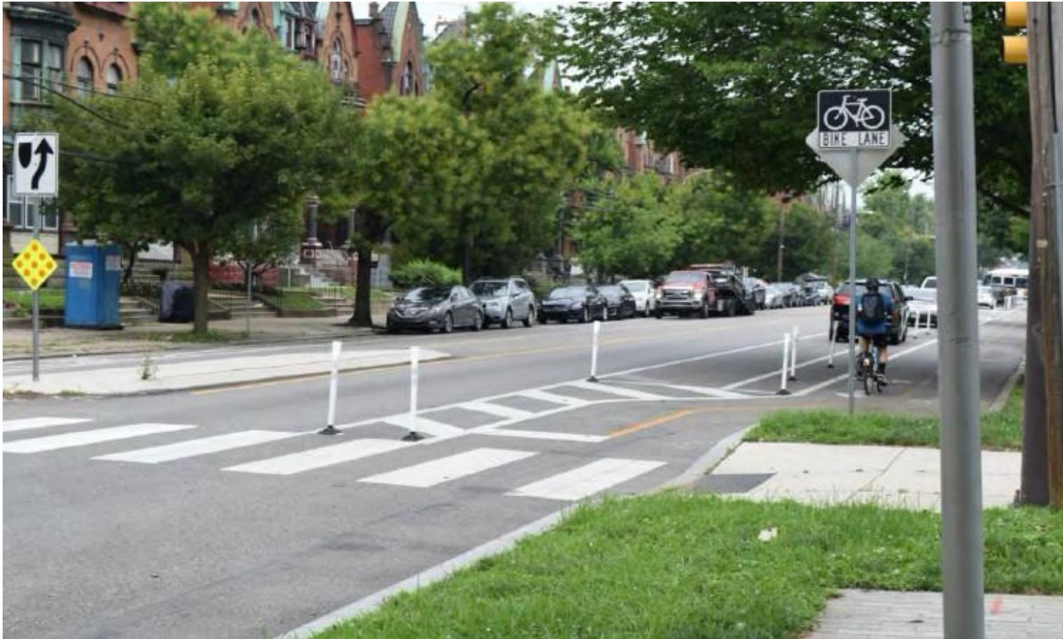
*Photograph 1:* Parkside Avenue, Philadelphia - Improvements include striping, markings, flexible delineators and signage.
