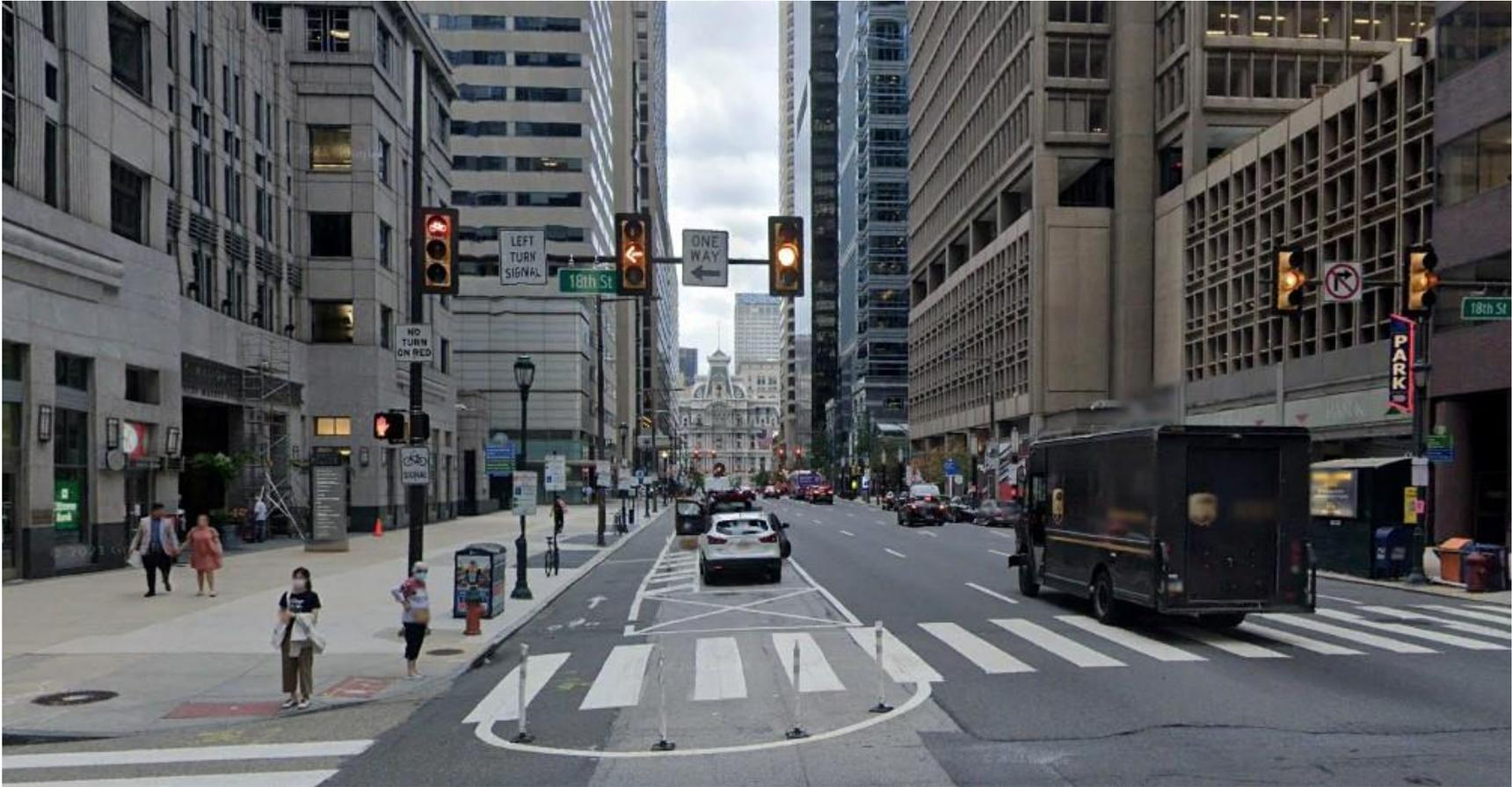
*Photograph 3:* Market Street, Philadelphia - Improvements include bicycle signal, flexible delineator post, painted buffer, and bicycle pavement markings.
