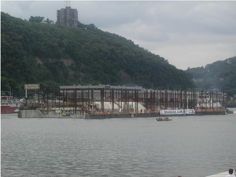
Figure 3 - Elizabeth Lock dewatered revealing its deteriorated condition
