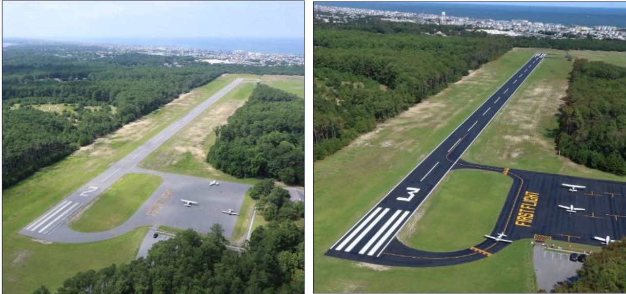
Before and after photos of a typical NC airport pavement maintenance project.
